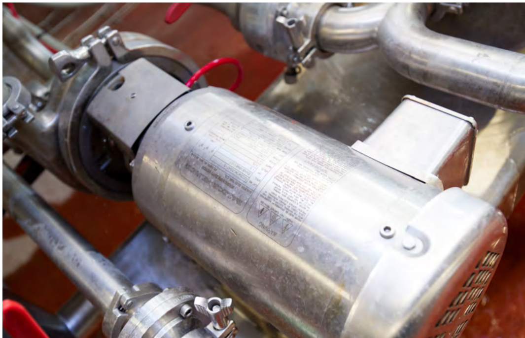
One of many Baldor motors attached to the McDonald Steel vat and tub brewing system at the Toronto-area Henderson Brewery.
