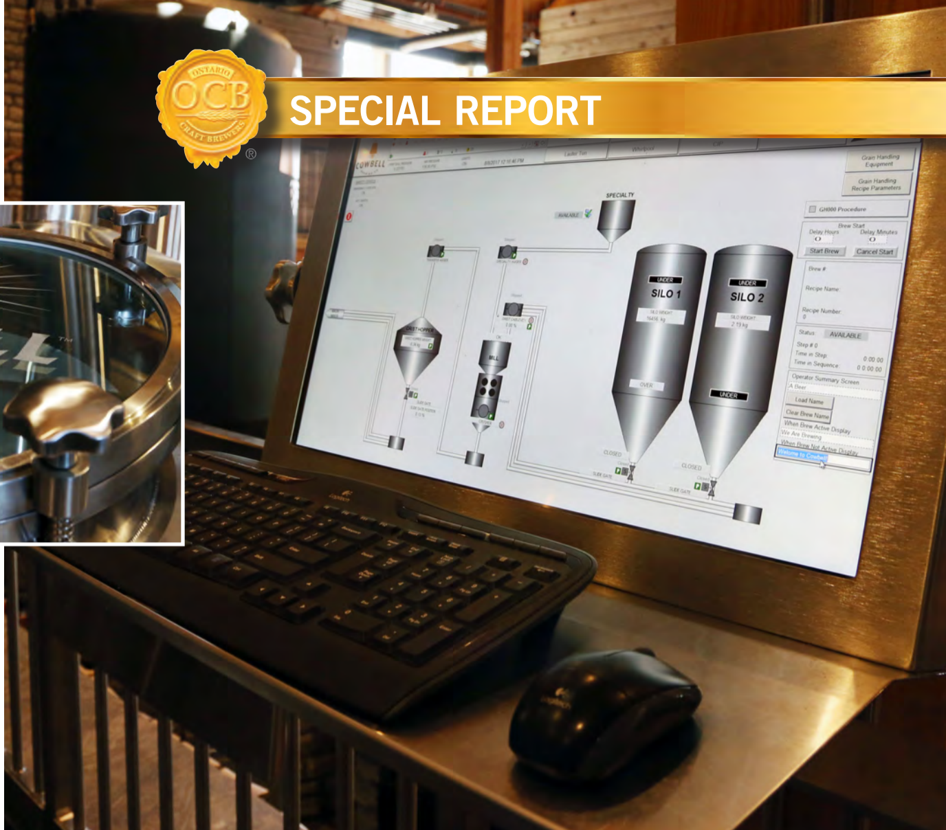
All the brewhouse operations are displayed and monitored in real time on a computer touchscreen interface via user-friendly icons and graphics to keep plant personnel constantly updated on the brewing process.
