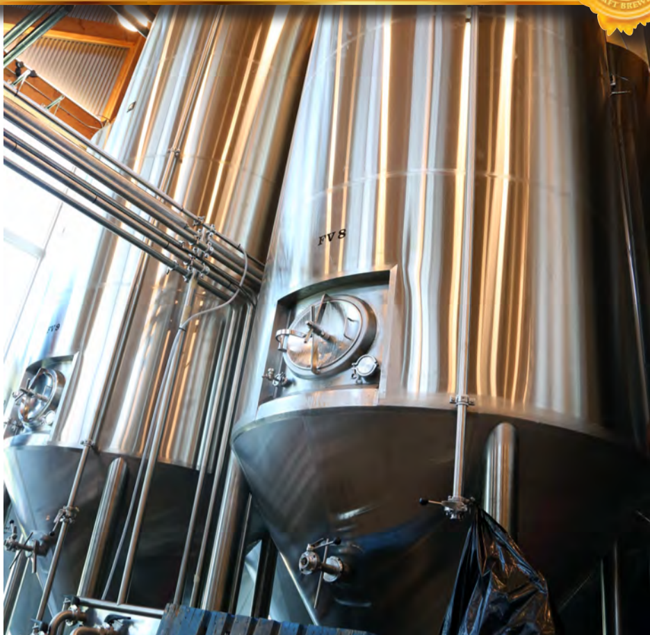
The Cowbell Brewing facility currently houses 10 large stainless-steel fermentation tanks to produce its growing range of beer products, with plans to add many more in coming years.
