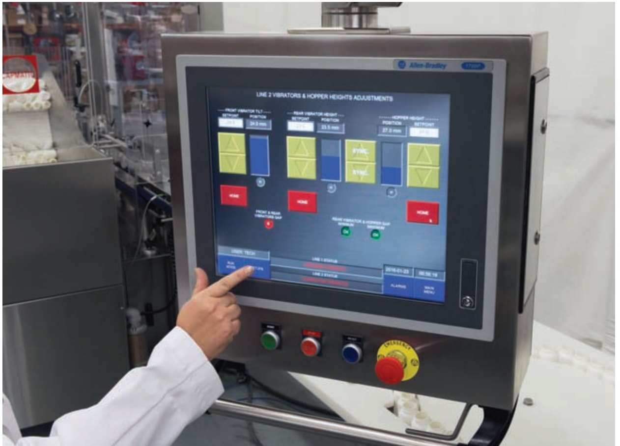
The Street Fighter uses the latest PLC (programmable logic controller) programming to ensure optimal process control.
